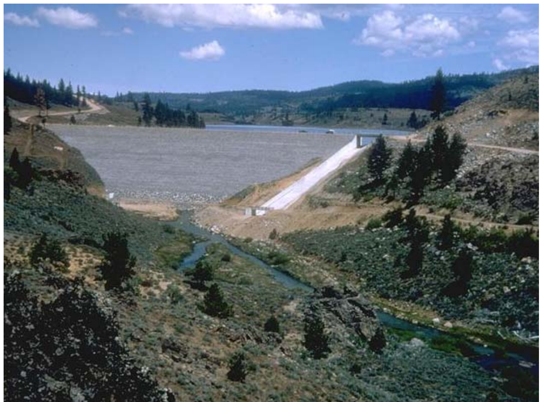
Figure 41. Photograph of dam and spillway (courtesy of California Department of Water Resources)
