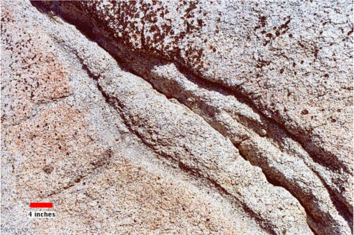
Fig. 1 Closeup of fracture in rock outcrop in the Tierra del Sol watershed.
