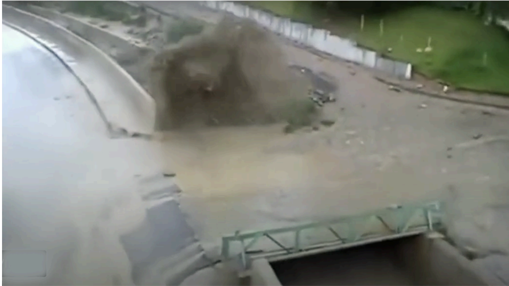
Fig. 4 Roll waves on the Huayñajahuira river channel, La Paz, Bolivia, on December 11, 2021.
