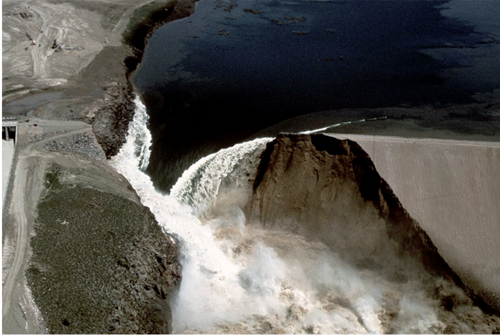
Fig. 1 Failure of Teton Dam, on the Teton river, in eastern Idaho, on June 5, 1976, clearly an example of a strongly attenuating flood wave.
