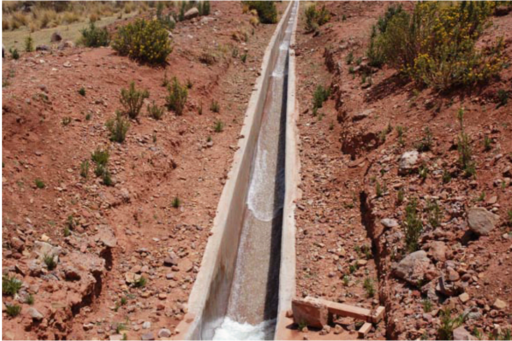
Fig. 3 A train of roll waves traveling in a steep irrigation canal, Cabana-Mañazo, Puno, Peru.
